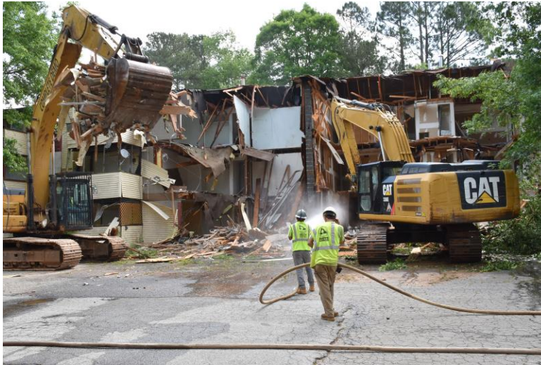
The county demolished 56 units at Brannon Hill Condominiums.
