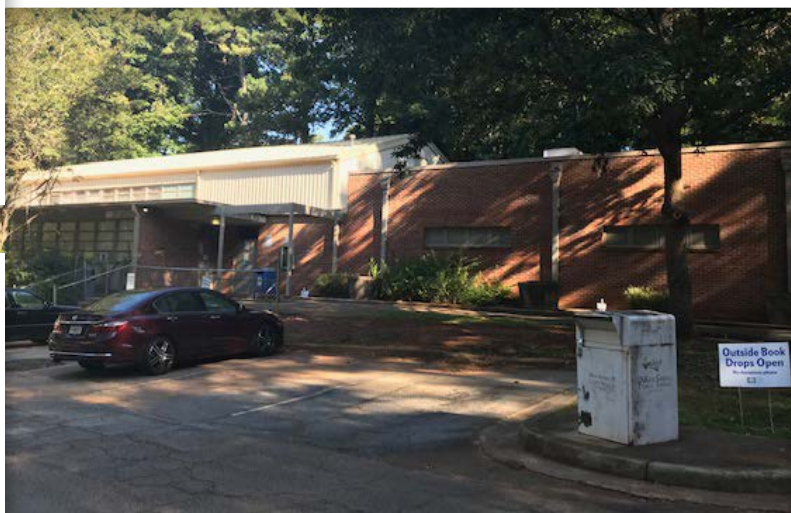
The more than 50-year-old building that housed the former Tobie Grant Recreation Center and Library
