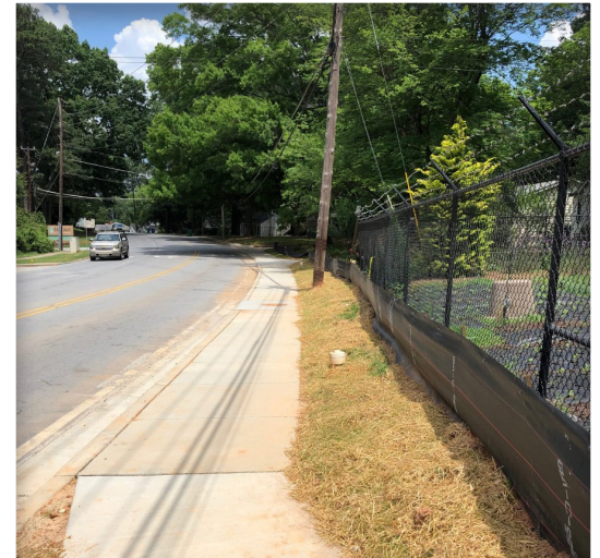
SPLOST-funded improvements made to the sidewalks at North Druid Hill Road and Valley Brook Road. Work is underway to transform the corridor into a multimodal-friendly complete street supporting various uses.
