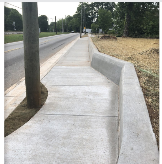
The first community meeting in May heard several concerns from residents and drivers. Top traffic concerns were congestion in the corridor, speeding, and safety. Our goal is to improve major intersections from an operations standpoint, reduce crashes, and increase pedestrian safety.
